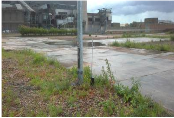
Photograph No.441 – Test location - Lamp Post.
