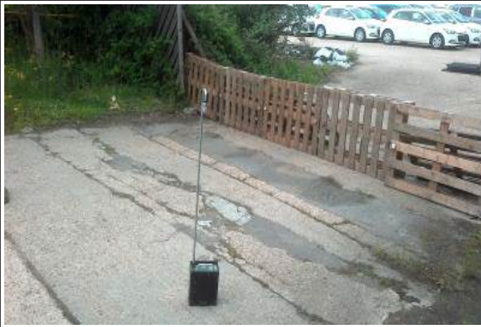
Photograph No.445 – Test location - Car storage entrance.
