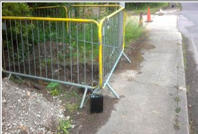
Photograph No.444 – Test location - Utility Excavation.
